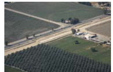
Aerial view of early construction on Hanford Expressway.
