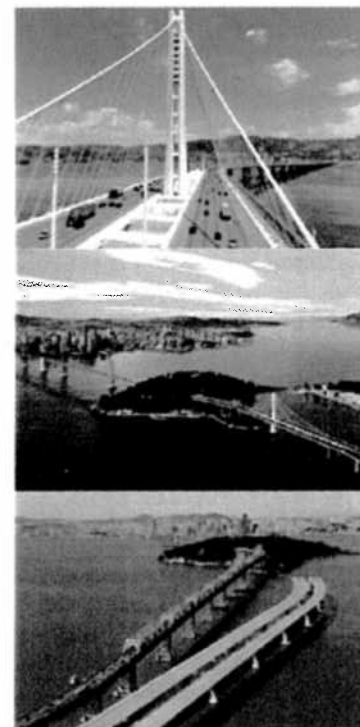
"Today we celebrate another impressive engineering and construction milestone in the ongoing seismic retrofit of one of the country's most vital bridges," said Dale Bonner, Secretary of the California Business, Transportation and Housing Agency. July 2010
