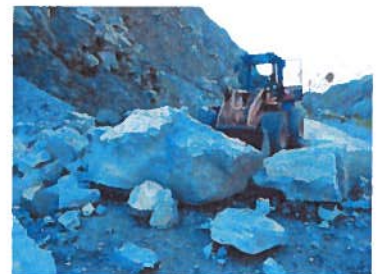
Below: Clearing rock fall on State Route 178 in the Kern River Canyon.
