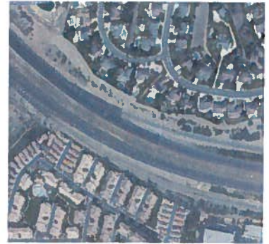
State Route 73 Paving Project
